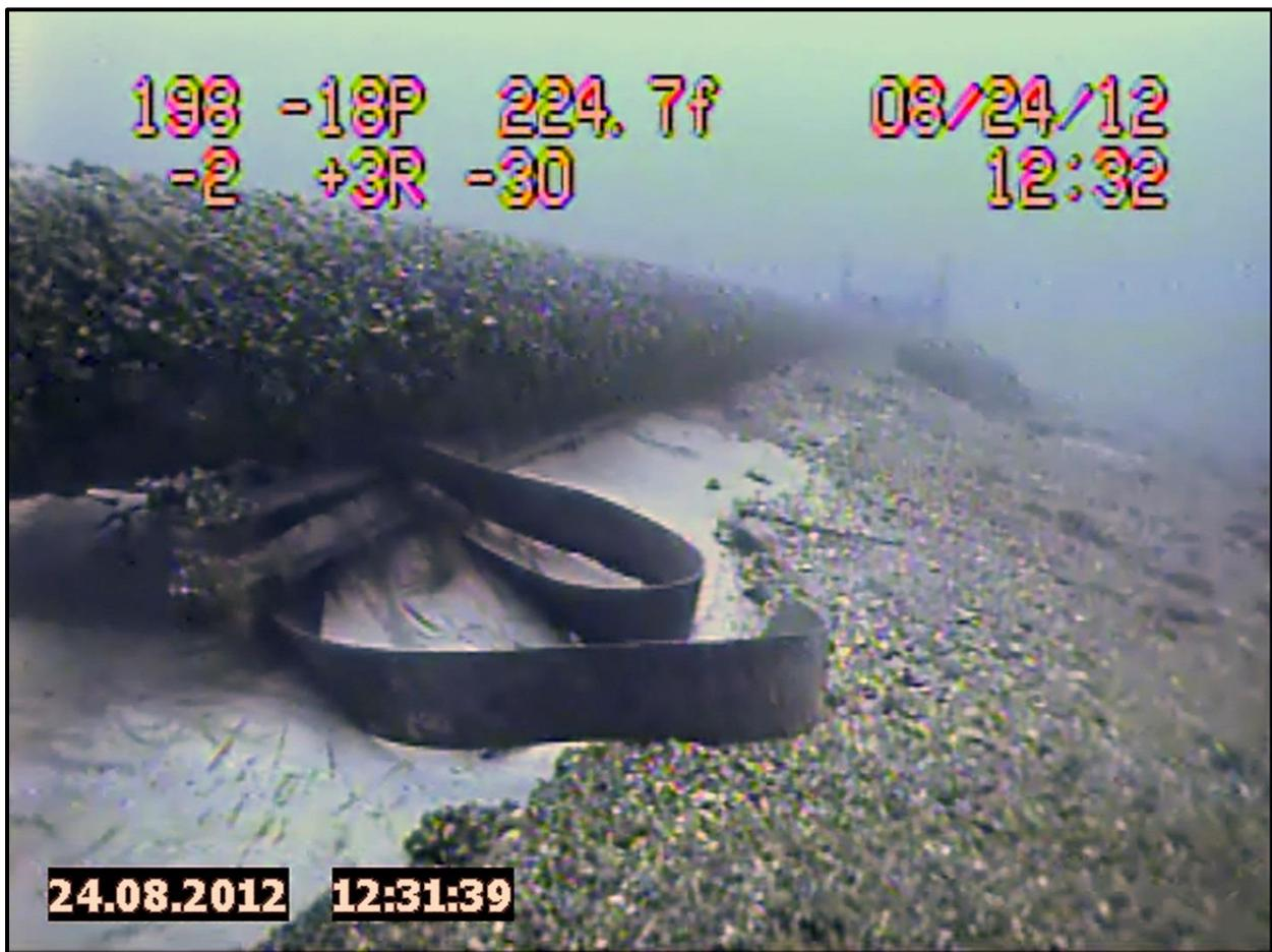
Figure 5 Broken Lifting Strap around West Leg from 2012 Enbridge Inspection Video
